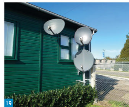
Fig. 15: The QO-100 voice SSB station. Fig. 16: Las Sanduly M0BOY demonstrates interactive digital amateur television reception. Fig. 17: SteppIR antenna. Fig. 18: 2m/70cm steerable dipole. Fig. 19: Satellite dishes for QO-100 reception and voice transmission.
